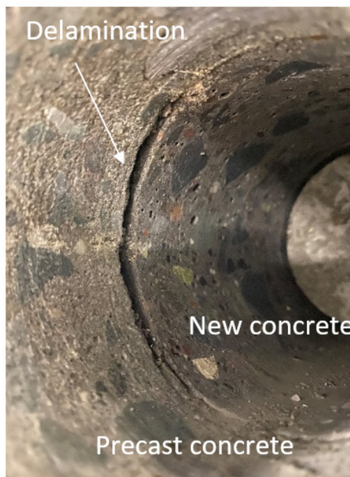
Hole in element. The delamination between the precast element and the new concrete can clearly be seen.
