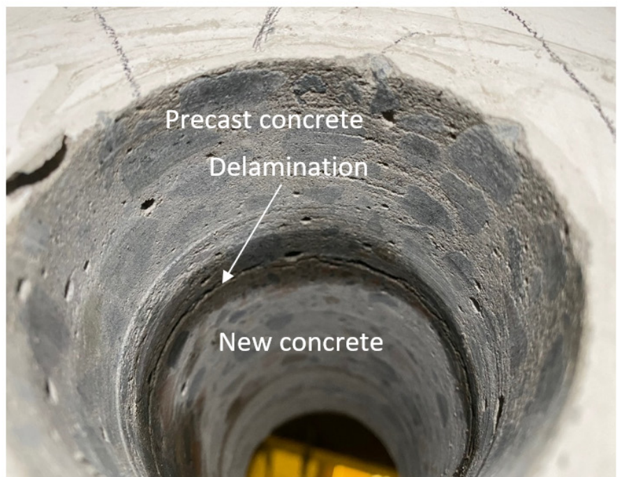
Hole in element. The delamination can clearly be seen between the precast element and the new concrete.
